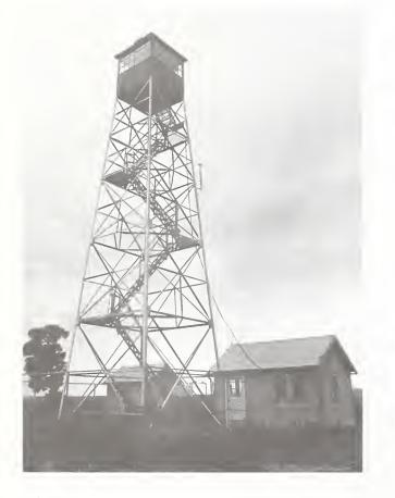
Figure 211. Bluewater lookout (either an Aermotor LX-24 or International Derrick) cabin, and storage shed.
